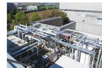
System using renewable thermal energy
