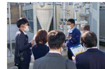
Reporting the launch of the verification test to the parties concerned
